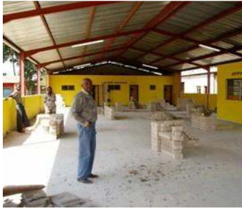
A interior of a partly finished 'health centre' contracted by a Chinese Company in Lusaka, Zambia
