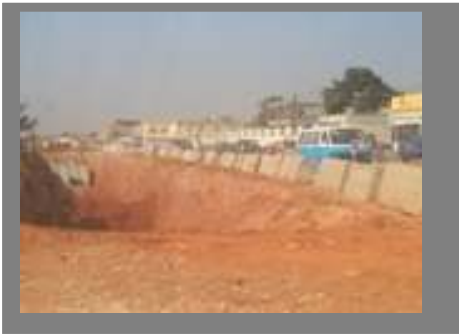
Road Rehabilitation in Luanda, Angola
