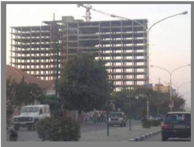
Justice palace under construction, Luanda
