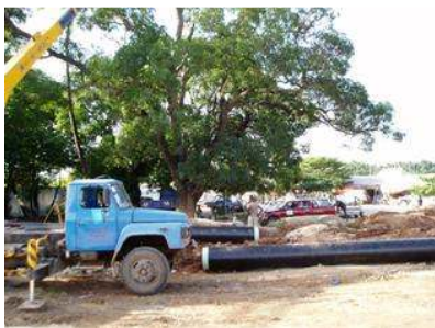
Construction site in Dar-es-Salaam, Tanzania
