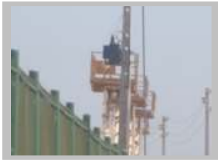
Construction Towers, Luanda, Angola
