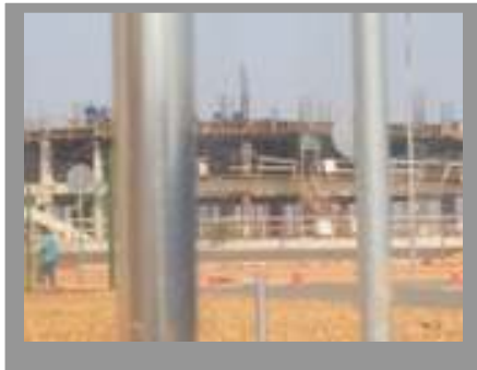
Construction at Futunga, Angola Sonangol Project
