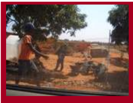
Construction workers on site outside Luanda
