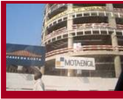
Construction site in Luanda sporting signboards of Portuguese construction companies
