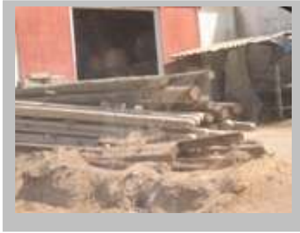
Construction site in Luanda, Angola
