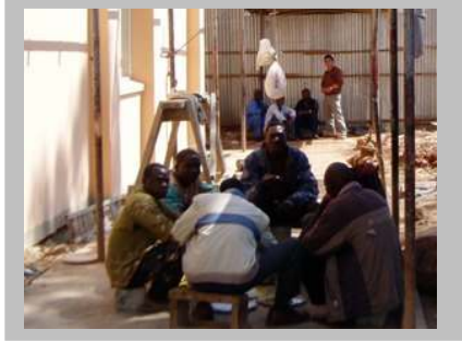
Group of Construction workers on site in Lusaka, Zambia
